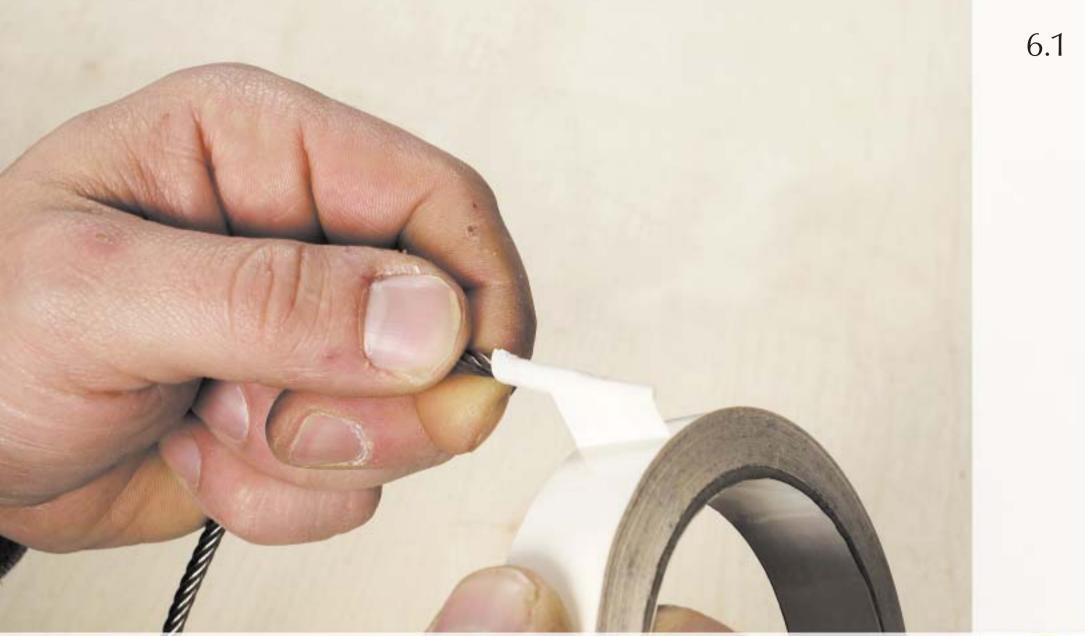
Wrap the end of the wire with insulating tape.
